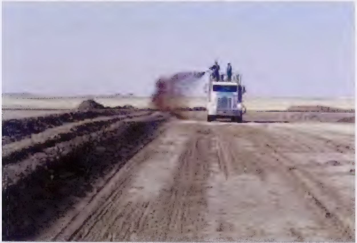
Photo 26 Applying soil tackifier to prevent wind erosion
